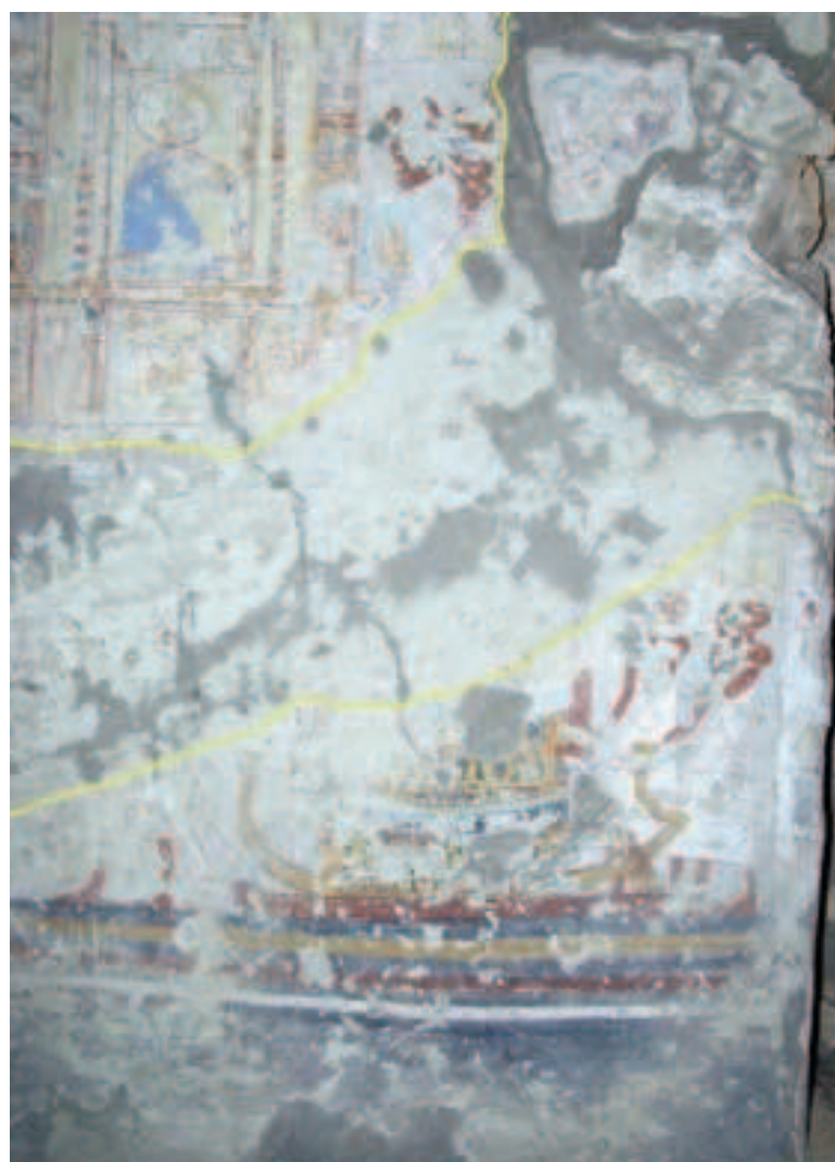
Fig. 131 - Sloping strip of muddy water erosion on the painted decoration of chapel “A” (TT 14).
