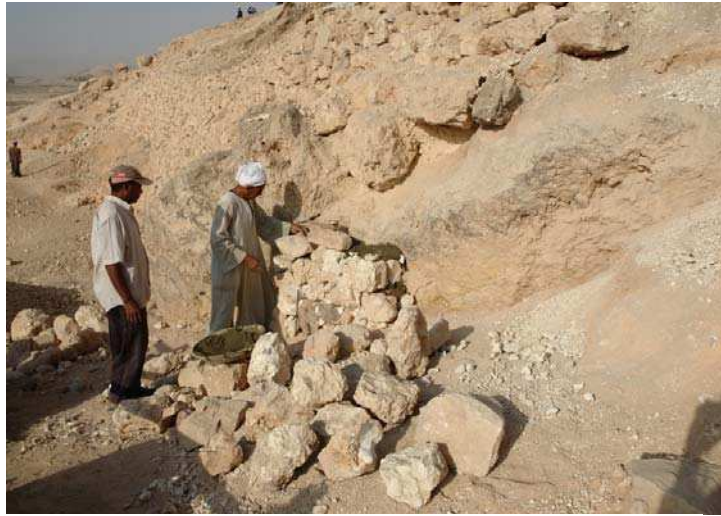
Fig. 8: Restoration and consolidation of the retaining wall
